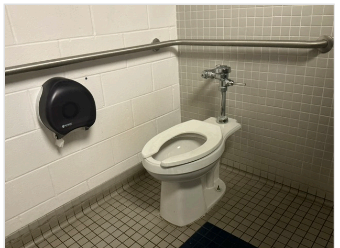
TOILET STALL OVERVIEW
