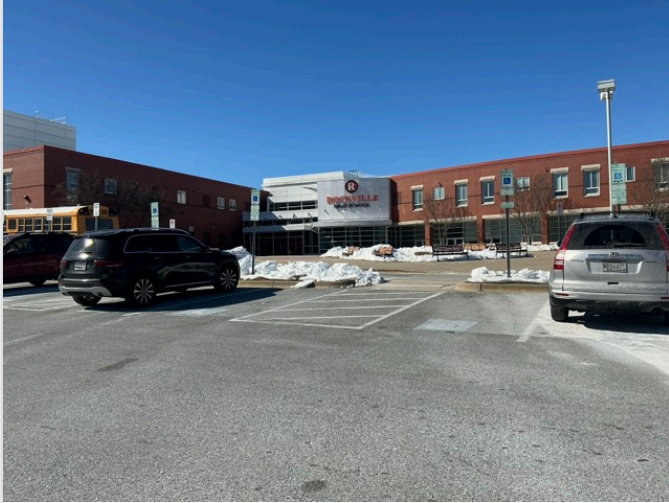
OVERVIEW OF ACCESSIBLE PARKING AREA
